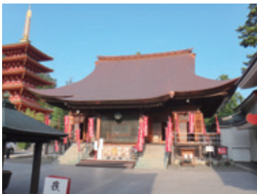
Fudo-do Hall of Kongo-ji Temple (Courtesy of the Japanese Association for conservation of Architectural Monuments)
